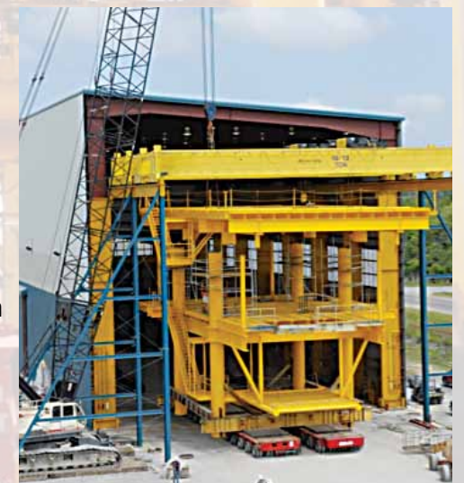
28,000 square-foot fabrication facility
